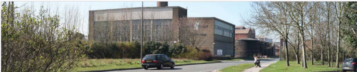
2. Looking south-west towards the existing 'gateway' to Selby past BOCM PAULS mill along Barlby Road
