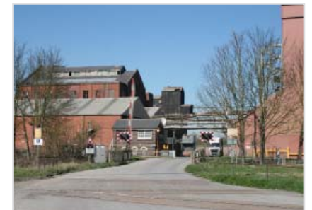
6. Looking north to the railway level crossing
