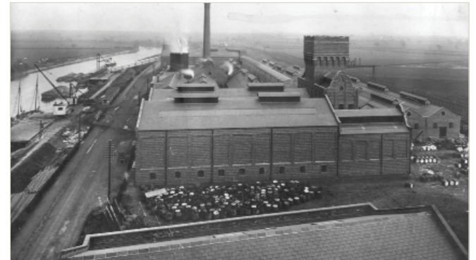
Pre-1913 BOCM PAULS mill looking east with Barlby Road shown on the left
