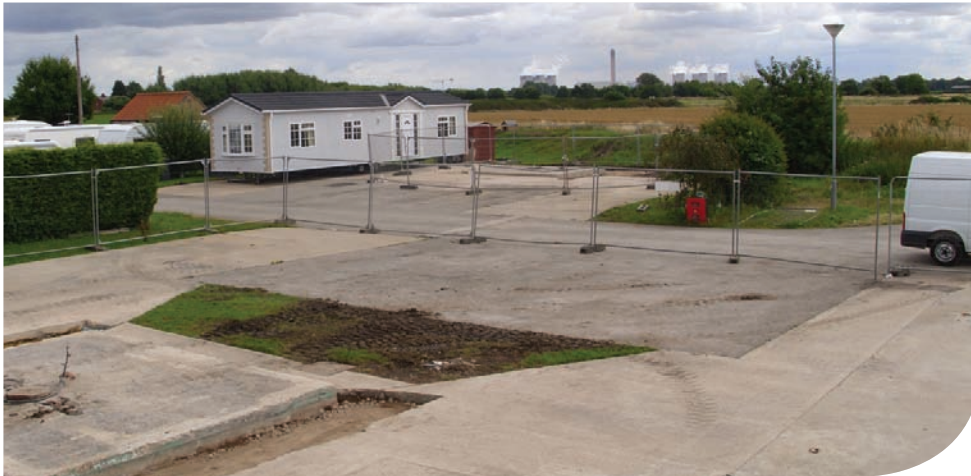
Burne Gypsy and Traveller site, Selby, ready for construction.
