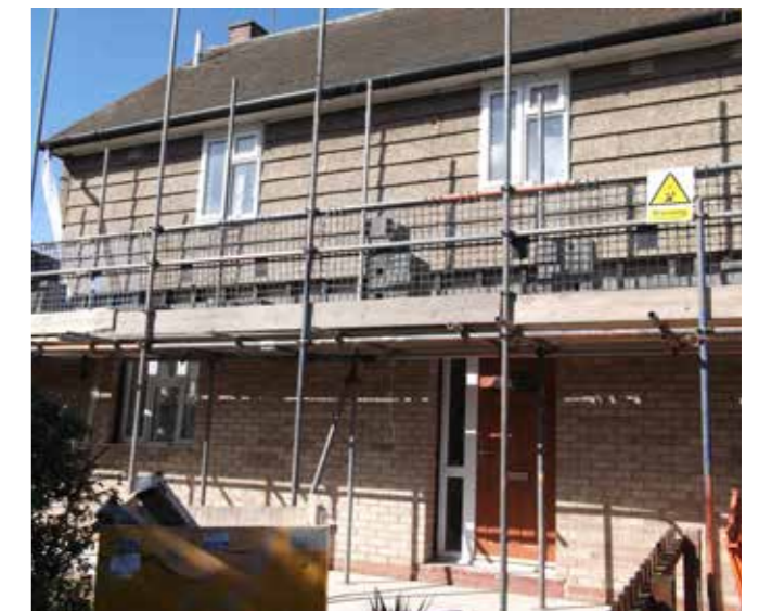
Renovation work at Airey homes.
