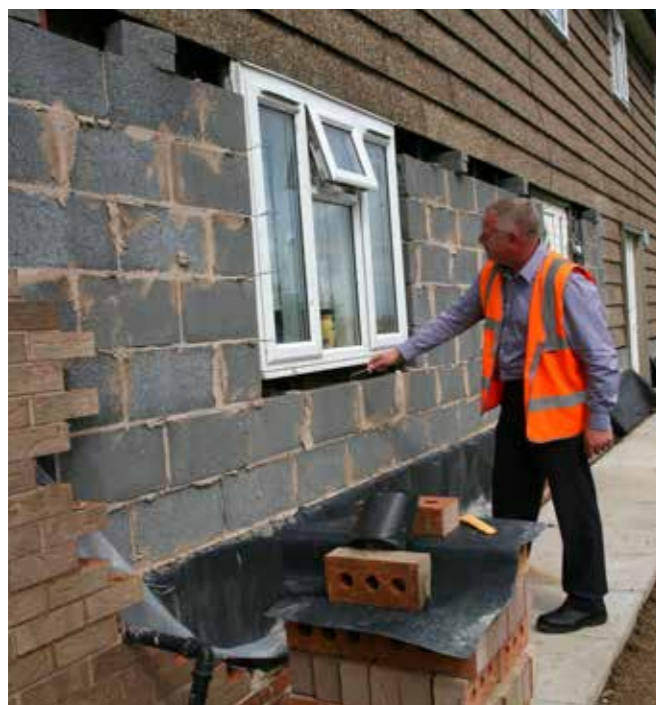
Checking the refurbishment work at Airey homes.
