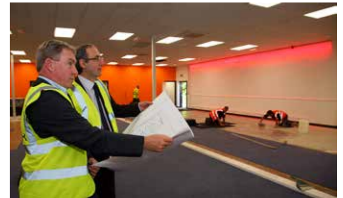
Checking progress at Profiles.
