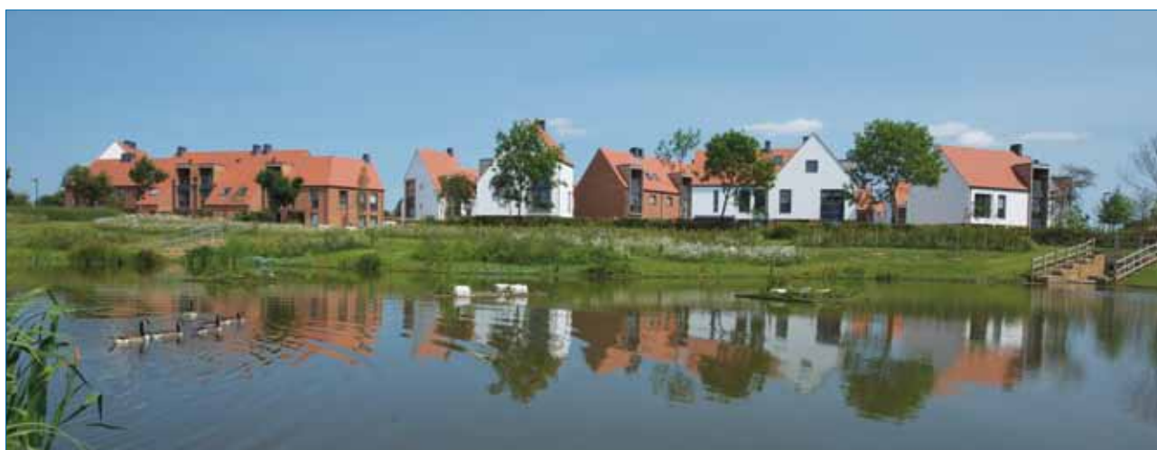
Derwenthorpe housing development
