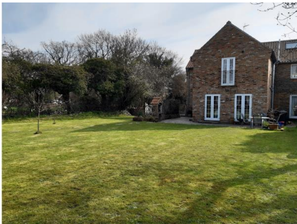
View looking east across garden of Jubilee Cottage
